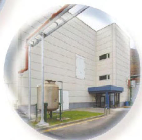
Capsulation facility (Ueda Plant)
